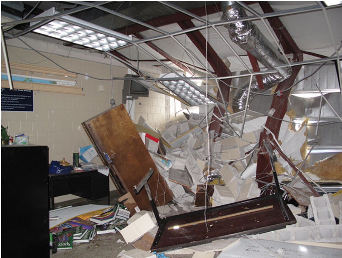
Figure 7: Re-cover roof structure failure—interior
